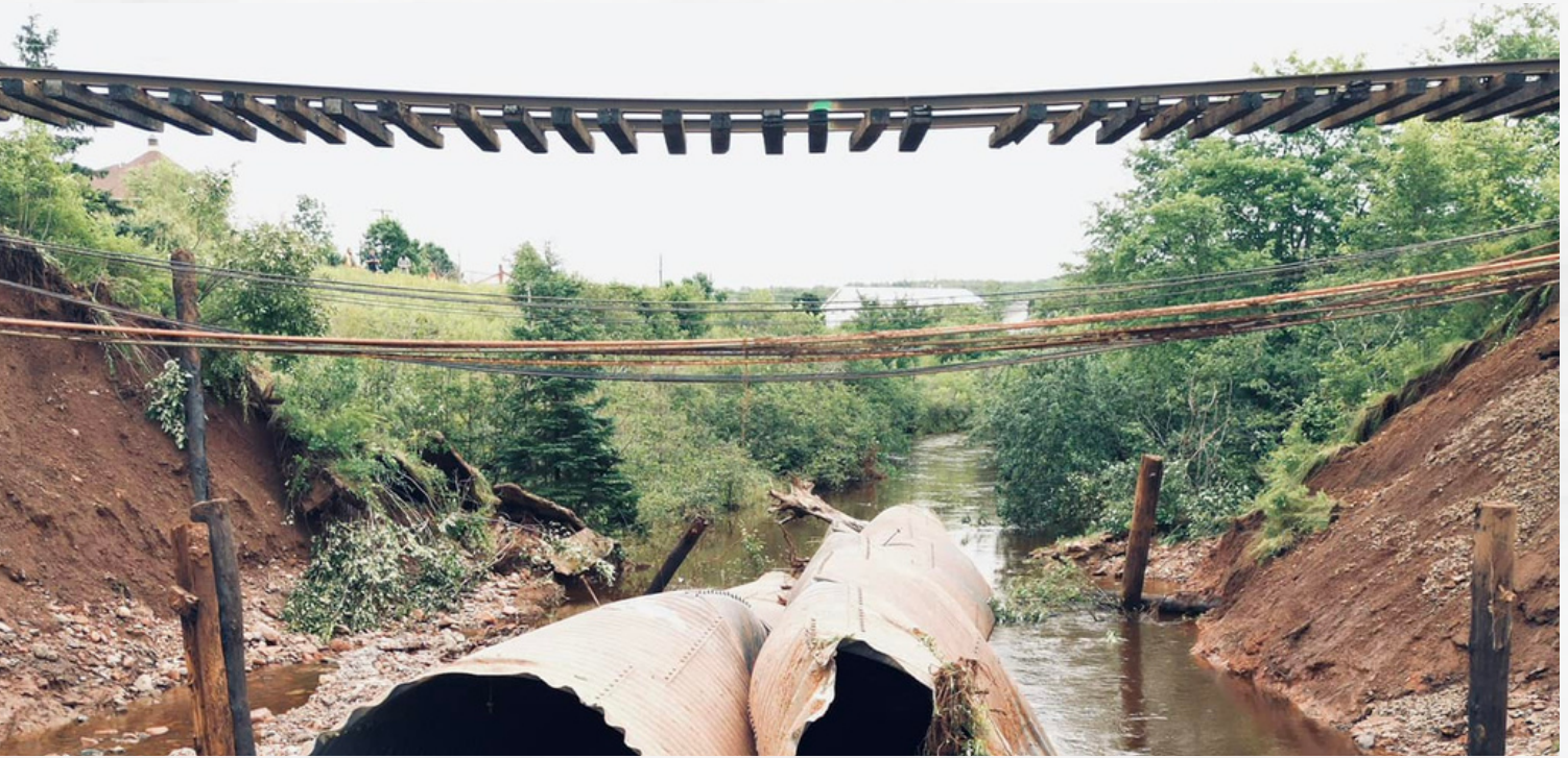
The devastating late July rainstorm affecting Colchester and Cumberland counties, clearly illustrates how quickly Nova Scotia could become an island. This Shaun Lowe Photographic image depicts remains of the CN mainline in Millbrook, near Truro. All rail transportation to-and-from the Port of Halifax was suspended until massive work was completed to reconnect the line. A similar nightmare would occur should the Isthmus of Chignecto dikes be breached, as water levels continue to rise due to global warming.
